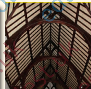
Hammer Beam Roof
