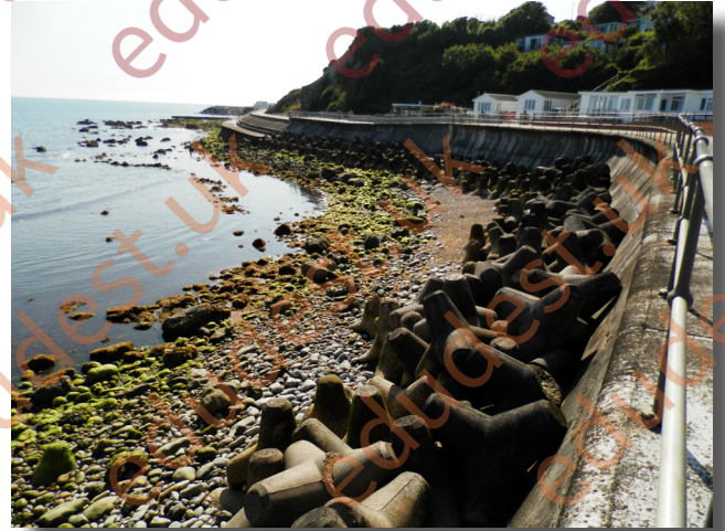
Concrete steps and rock armour at Ventnor Beach
