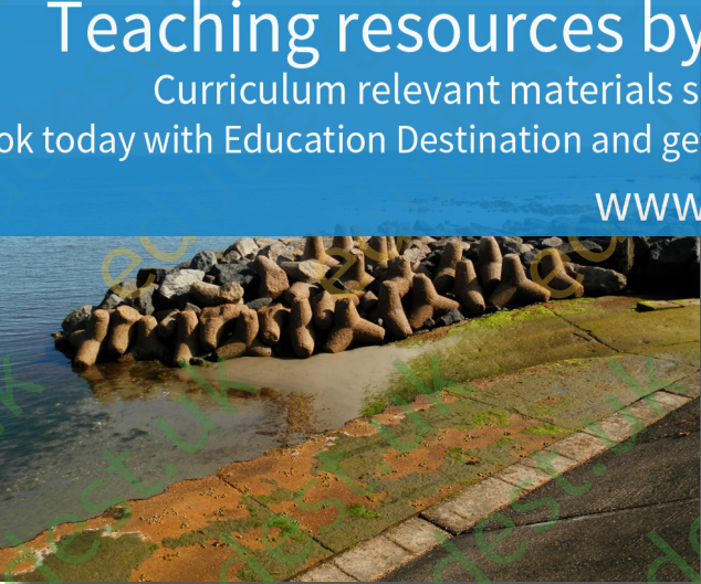
Rock/tetrapod breakwater at Wheeler's Bay
